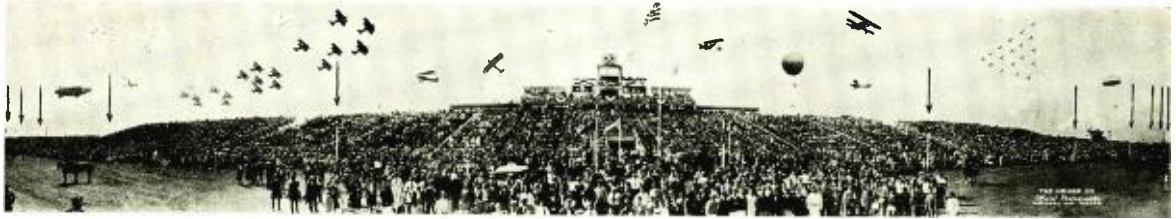
Loudspeaker installation in stands 3000 feet long, at National Air Races. Arrows indicate locations of loudspeakers.
